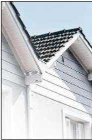
A roof with SOFFITS
