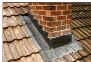
LEADWORK on a roof
