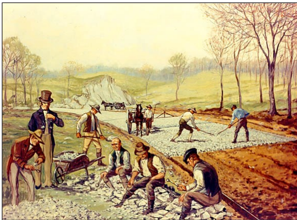
Road makers breaking stones to precise specifications, 1823
