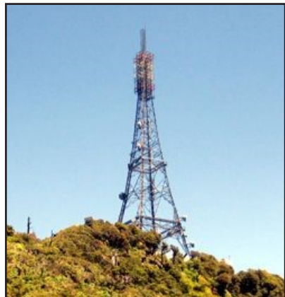
Mt. Te Aroha's mast
